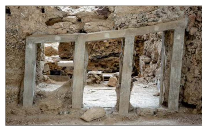
Polythyron in the ground floor of the east wing of Xeste 3. Its frame, distorted due to the decay of the timbers, was replaced with reinforced concrete in the course of its excavation.
