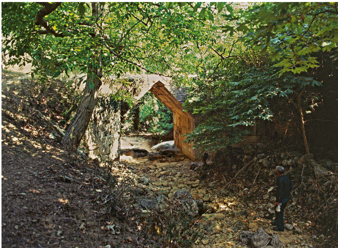
View of the Hellenistic bridge of Eleutherna.
