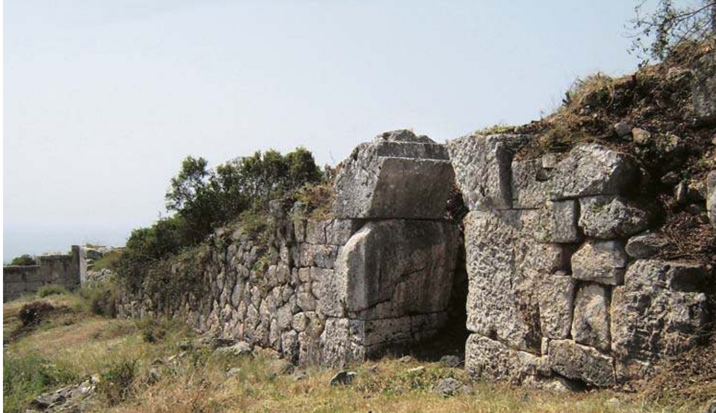
Typical section of the defensive wall of polygonal masonry with a gate in its archaic phase, the building of which is usually attributed to the tyrant Polycrates. The walls of this phase were demolished under the terms of the treaty that followed the Samians' defeat by the Athenians in 440-439 BC.
